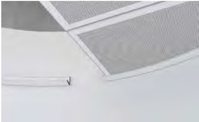
L-Wall Profile Concave (bent inside)
