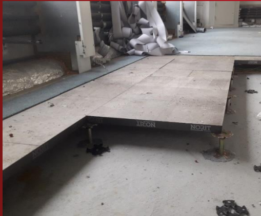
Panels in the refurbishment project
