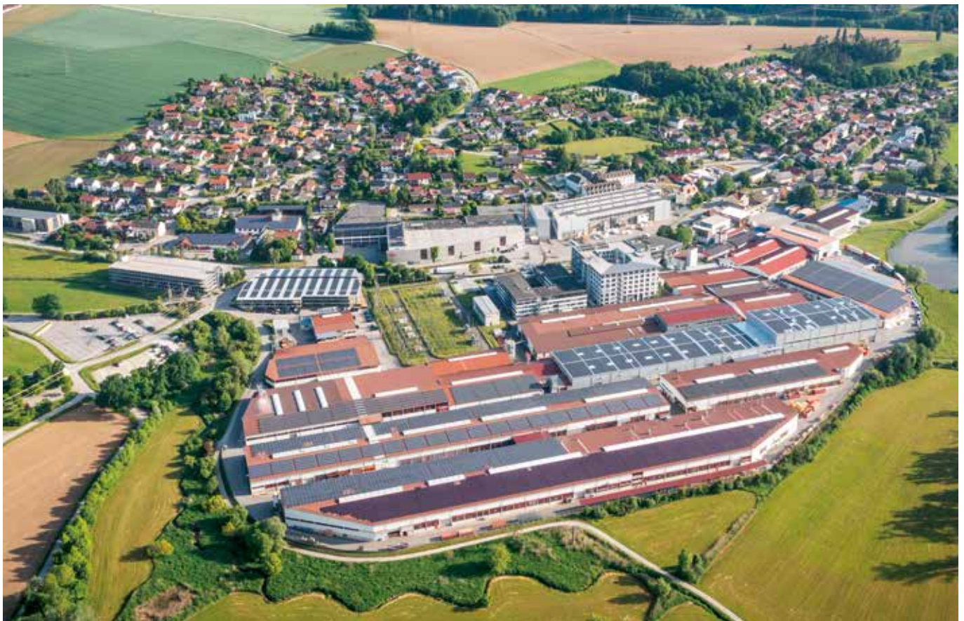
Lindner Group Headquarters Arnstorf, Germany
