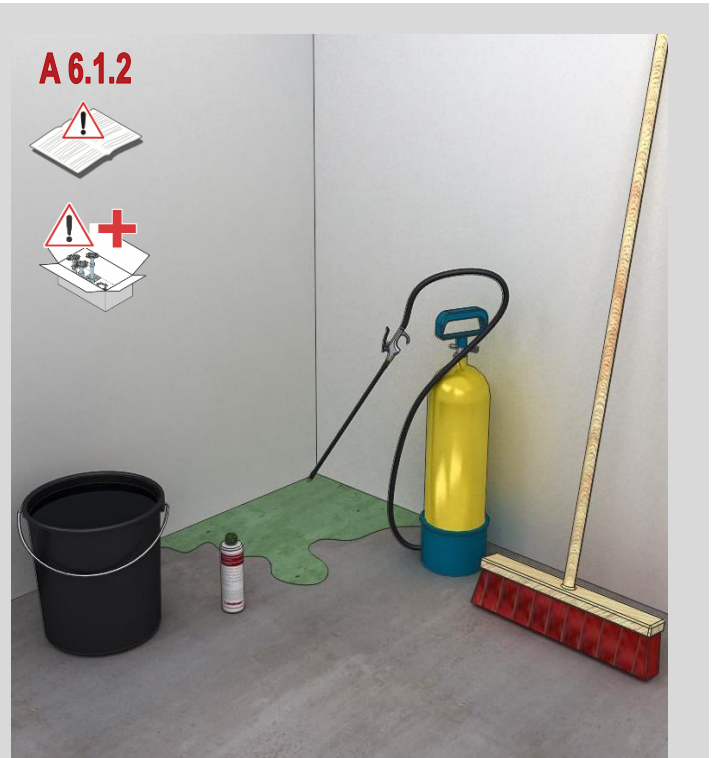
Picture 5 Application of the subfloor sealing
