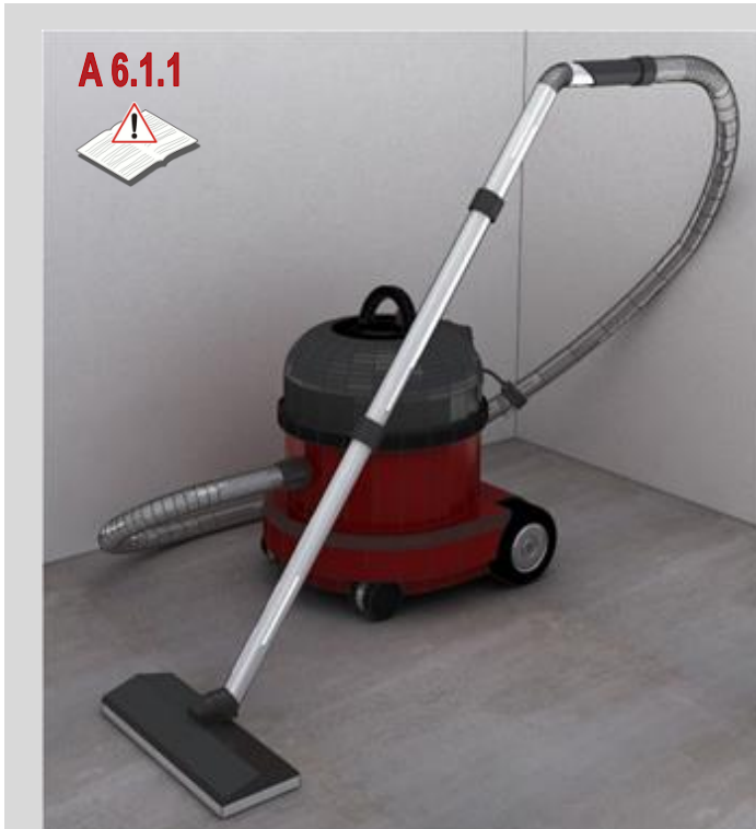
Picture 4 Cleaning of the subfloor
